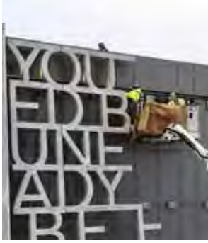
Photo, Envel Facade
